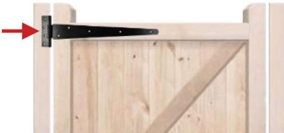
Remove gate and drill pilot holes. With two people, put the gate back on the packer and fit hinges to mounting posts. At this stage just use two screws per hinge so that you can check the gate swings freely before fixing the rest of the screws. Once done, remove bottom packer.
