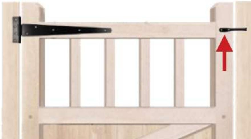
With the gate in the closed position, place the latch under the bar to check for position, mark holes, remove, drill pilot holes then attach with screws to post. Check the gate opens and closes securely. If needed adjust.
